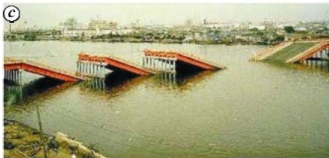
Figure 2. Failure of the Showa Bridge during the 1964 Niigata earthquake (NISEE 17 ).
